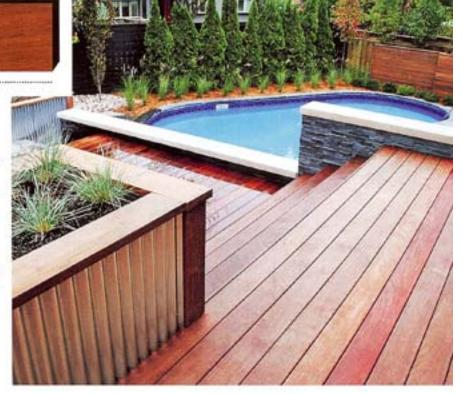
wood.com) is West Coast fir that is ACQ pressure-treated and then profiled, meaning grooves are placed into the surface of the wood to release the surface tension, making it less likely to split and crack.
