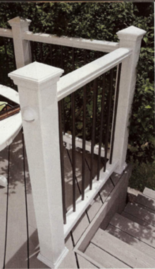
THE RAILING system (above) is covered in a low-maintenance, composite skin, but the structural integrity is provided by the inner, pressure-treated 4x4 post. The below-deck storage area is accessed via a hinged door built into the deck skirt
