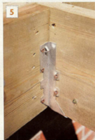
5. Galvanized joist hangers are the most secure way to fasten joists to the ledger board
