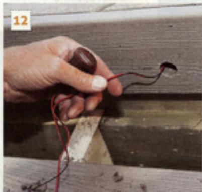
12. Small LED lights are set into the stair risers and will illuminate the treads to make evening entertaining safer
