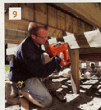
9. Extra bracing was added in the high-traffic area near the stairs
