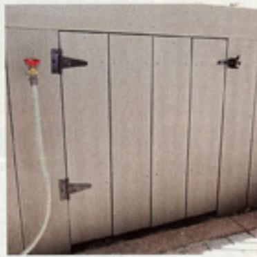
THE RAILING system (above) is covered in a low-maintenance, composite skin, but the structural integrity is provided by the inner, pressure-treated 4x4 post. The below-deck storage area is accessed via a hinged door built into the deck skirt
