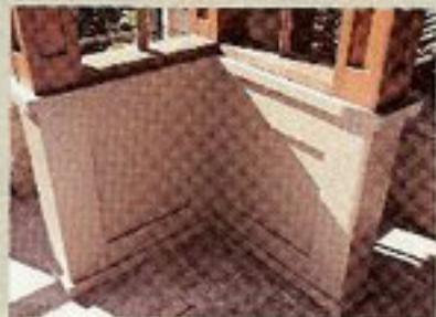
Start by preparing wood for the vertical side members (the stiles) and the wider horizontal members (the rails). The key is that all the parts be exactly the same thickness.
